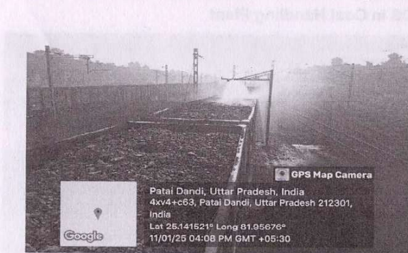
Figure: Pre-wetting of Coal Wagons
