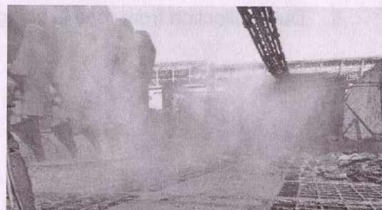
Figure: Water sprinkling in Wagon Tripler
