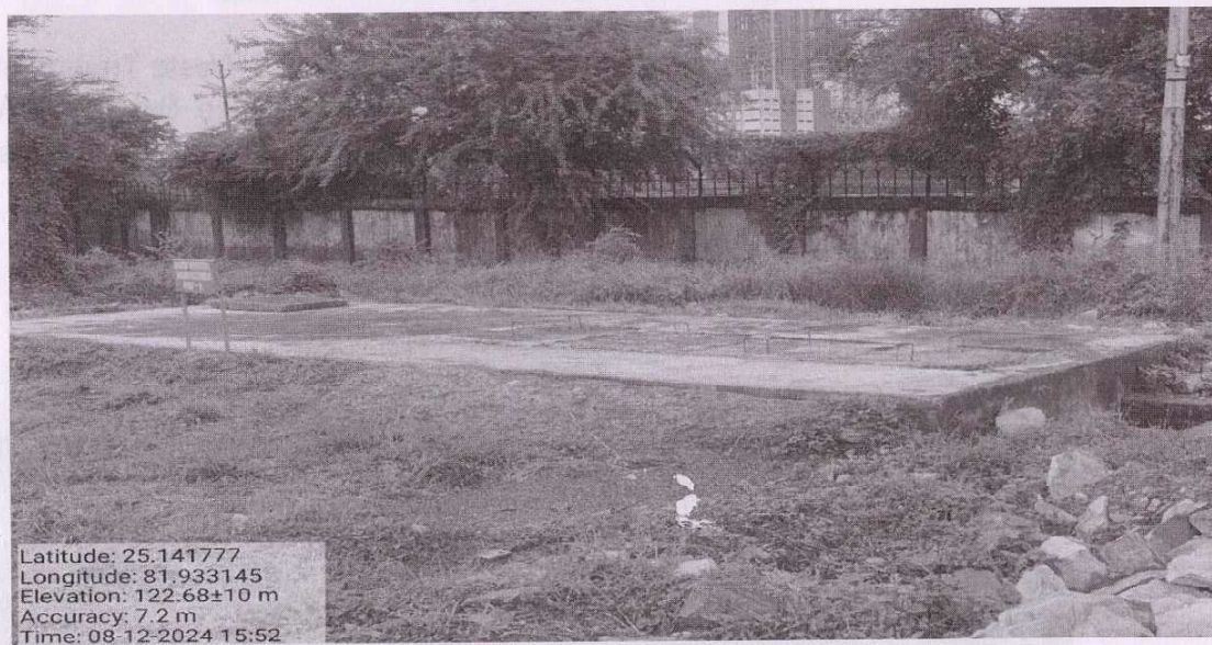
Figure: Rainwater harvesting pit: Township
